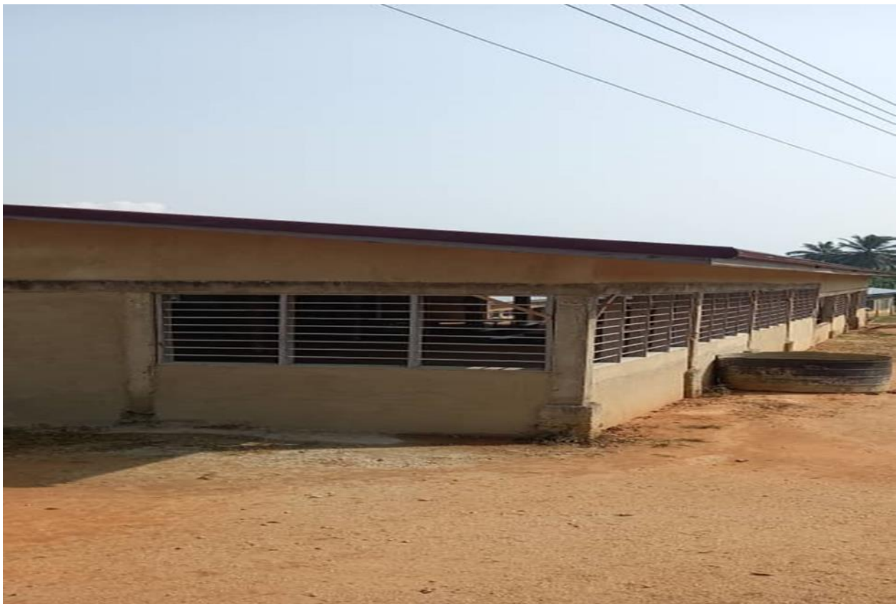
Super structure of Oguaa secondary Tech. school Dinning Hall Completed - DACF
