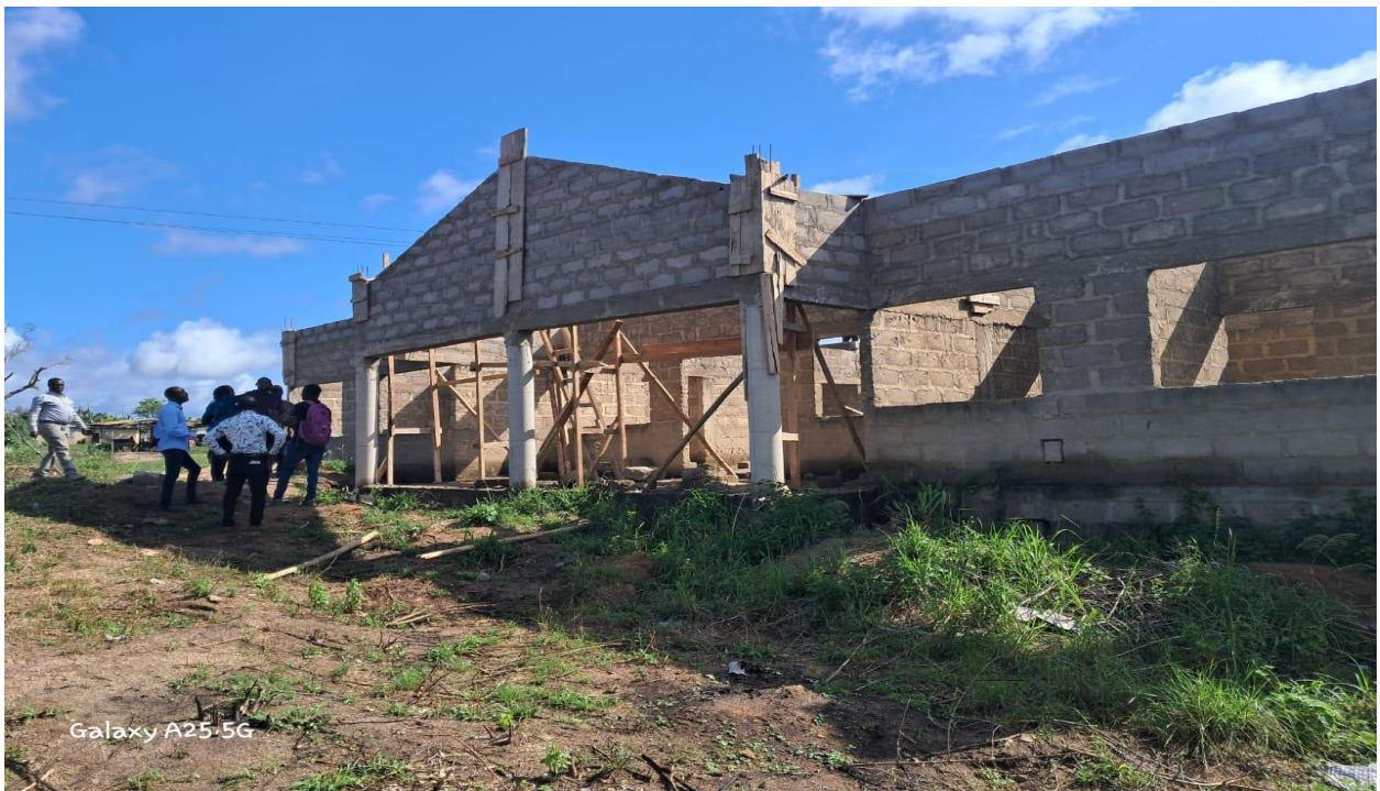
Super structure of police station at sewin completed
